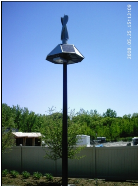
Vertical Axis Turbines on Street or Parking Lot Light
