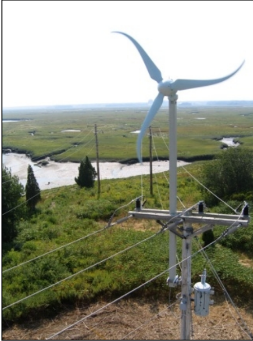
Horizontal Axis Turbine on Electrical Line & Street or Parking Lot light
