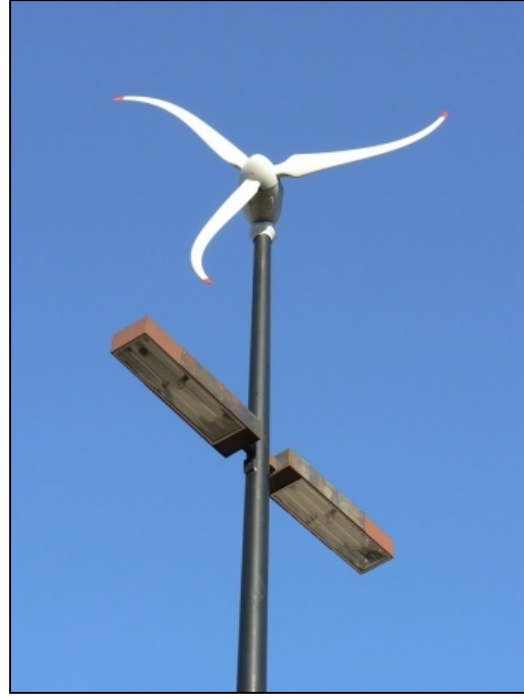
Horizontal Axis Turbine on Electrical Line & Street or Parking Lot light
